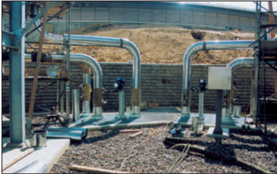
This vertical Porcupine retaining wall surrounds the exposed sections of the treatment plant constructed below the sight line of the surrounding area.
